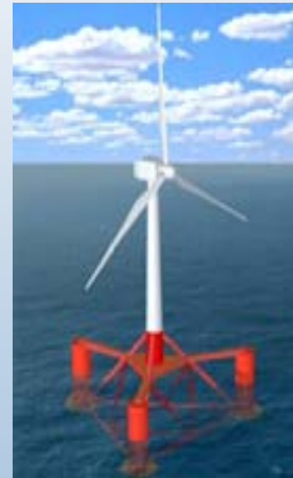
Wind Turbine on Dutch Tri-floater
